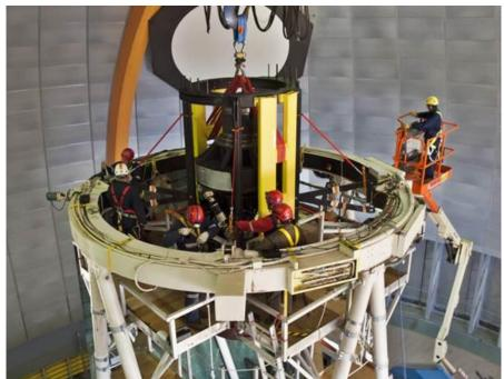
**Figure 12:** The new top end of the Blanco 4m telescope, during installation of the new prime focus cage to hold DECam.
